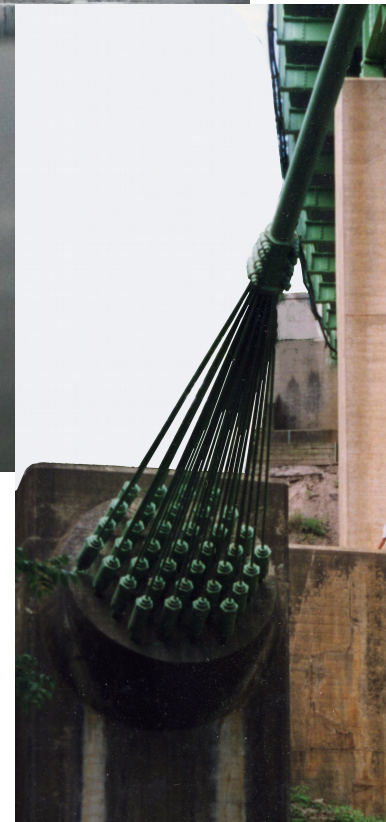
Typical suspension bridge cable ends
